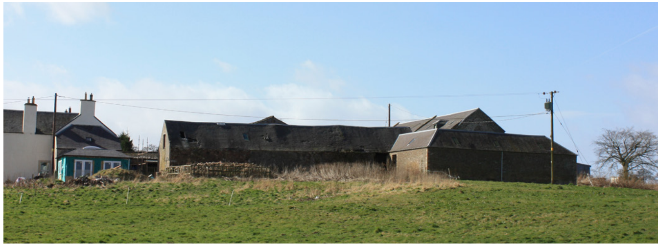
4. View of the Northern Edge of the adjacent buildings.
