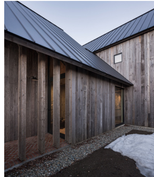
2. Precedent Image showing proposed combination of natural untreated timber cladding and standing seam roofing.
