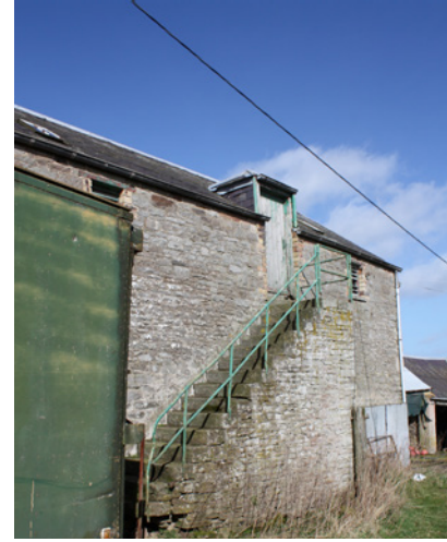
3. View of the west elevation of the existing building.
