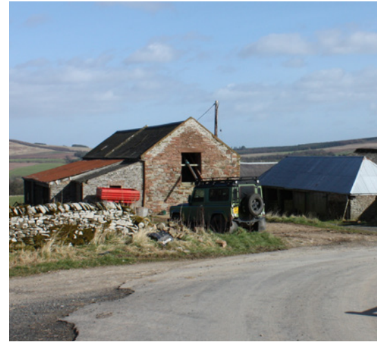
2. Photo showing rectilinear stone building and pitched roofscape.
