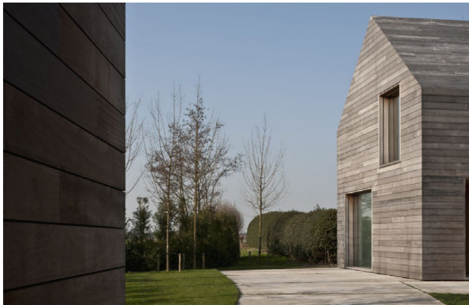
3. Precedent image showing use of contemporary detailing and fenestration proportions within traditional rural architectural massing.
