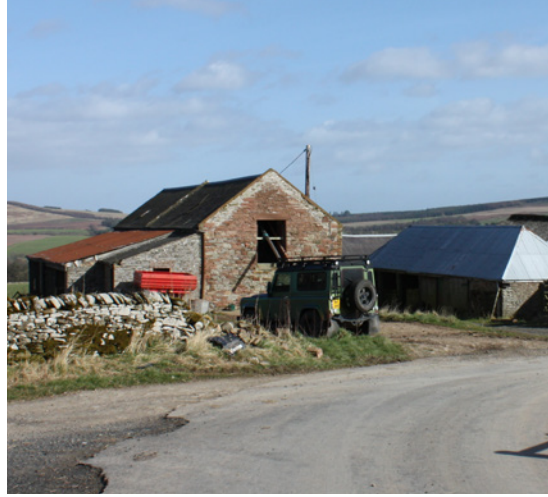
1. View of the South Gable of the existing building.
