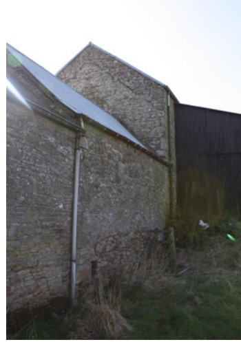
2. View of the North Gable of the existing building.
